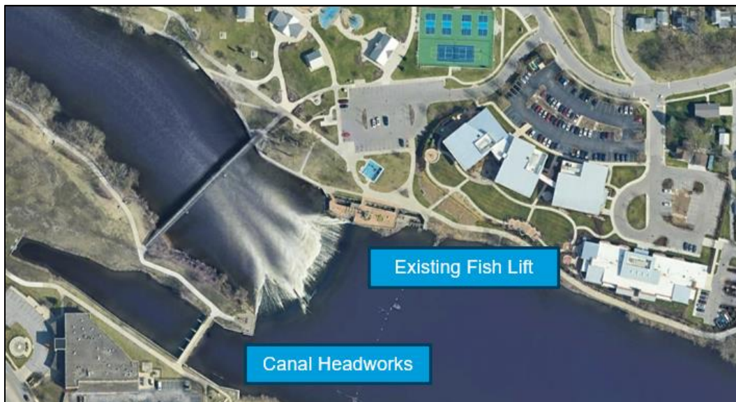
Figure 4: Aerial image of Mishawaka Fish Ladder in Indiana. Note the existing infrastructure that was discussed being used to integrate StreamDiver units.
