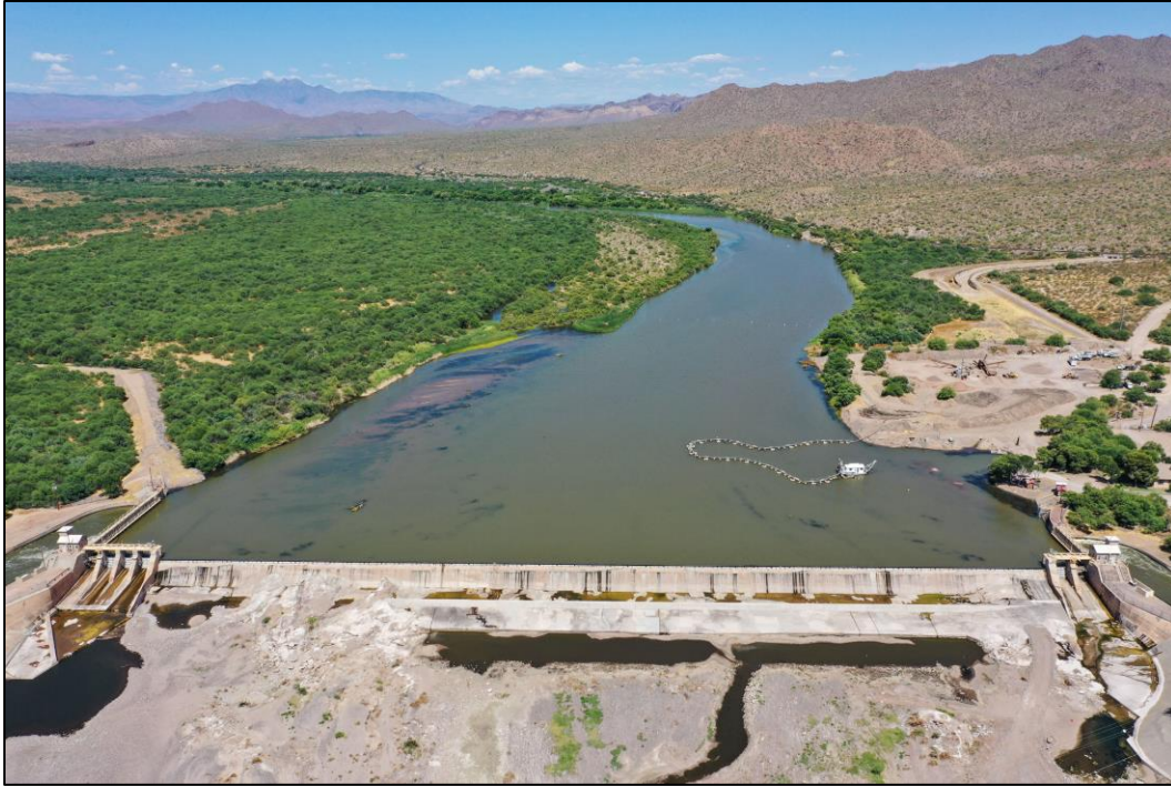
Figure 2: Granite Reef Diversion Dam full view. Note where water diverts into two canal systems, where we initially explored installing StreamDivers at.
