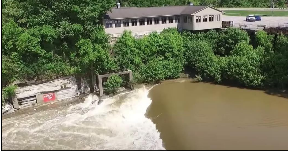
Figure 5: Existing flume structure visible along the bank of the river [5].
